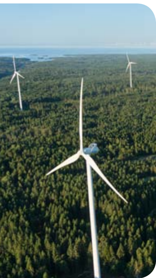
Vindpark Hakarp, Ronneby
