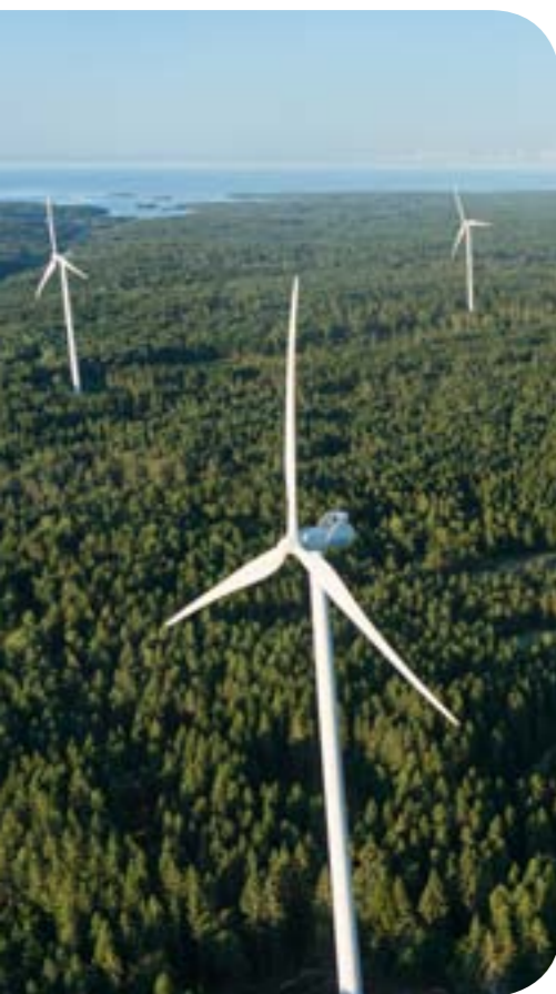
Vindpark Hakarp, Ronneby
