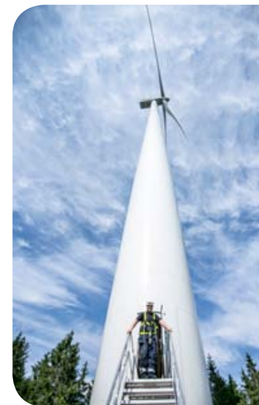
Vindpark Hakarp, Ronneby
