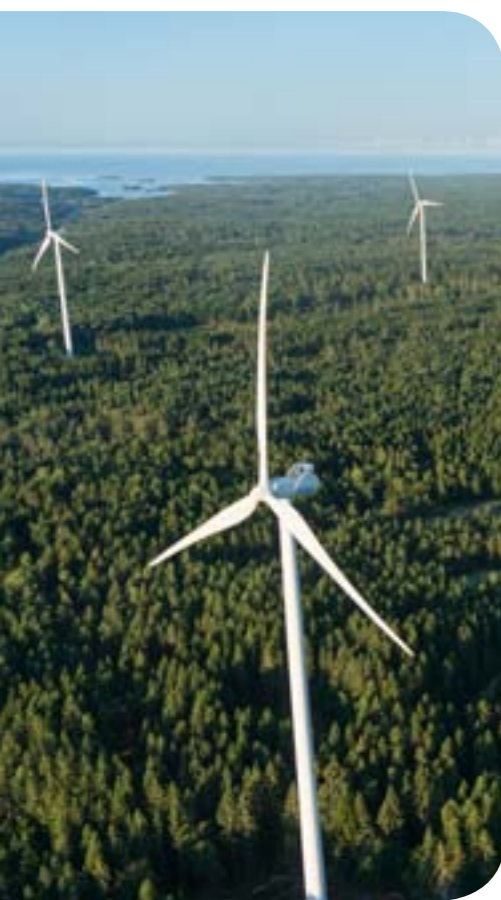
Vindpark Hakarp, Ronneby
